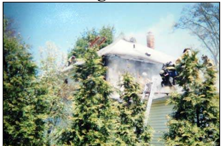
Heavy smoke at rear of the building made this an instant “Signal 10” working house fire as soon as the first volunteer arrived (Griffin photo)
