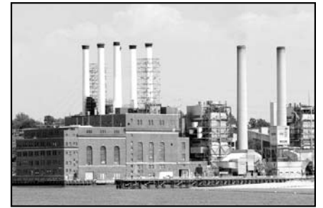
The Glenwood Landing power plant.
