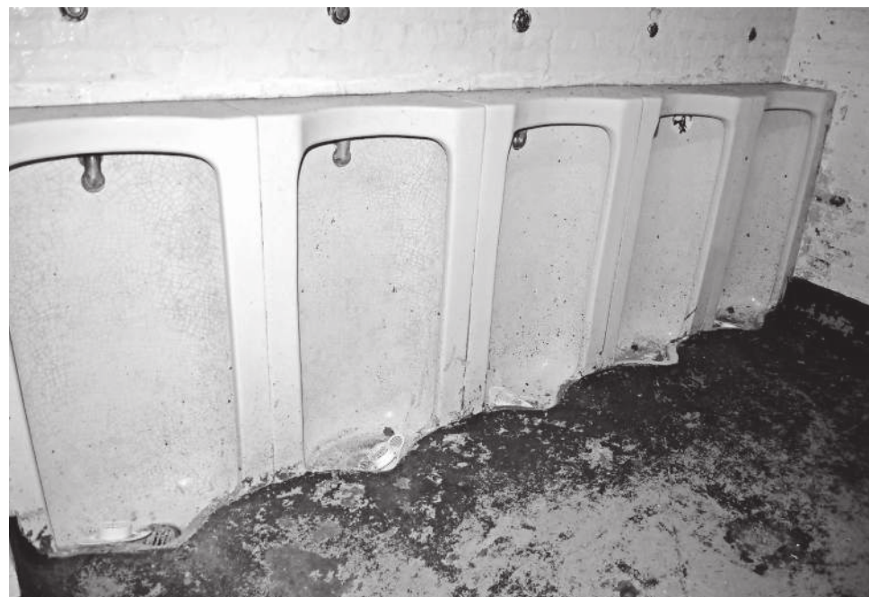
THE BATHROOM FLOORS will be replaced with heavy epoxy flooring.
