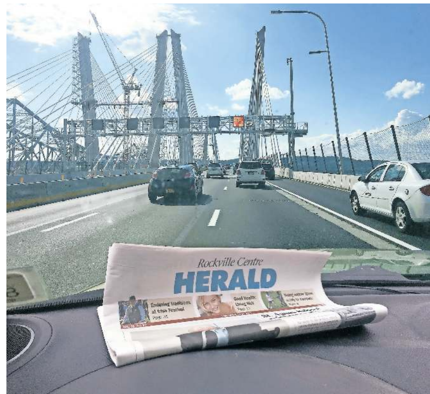
Making the long commute over the new Mario M. Cuomo Bridge — Tarrytown
