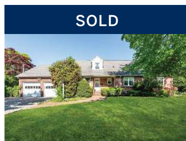
337 Carpenter Avenue, Sea Cliff, NY
